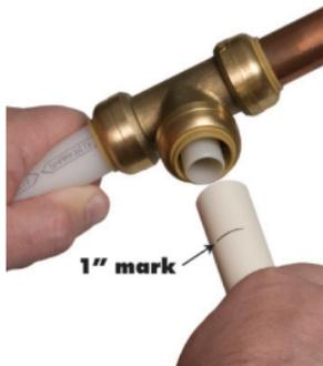
1. Insert the tube through the release collar to rest against the grab ring.
